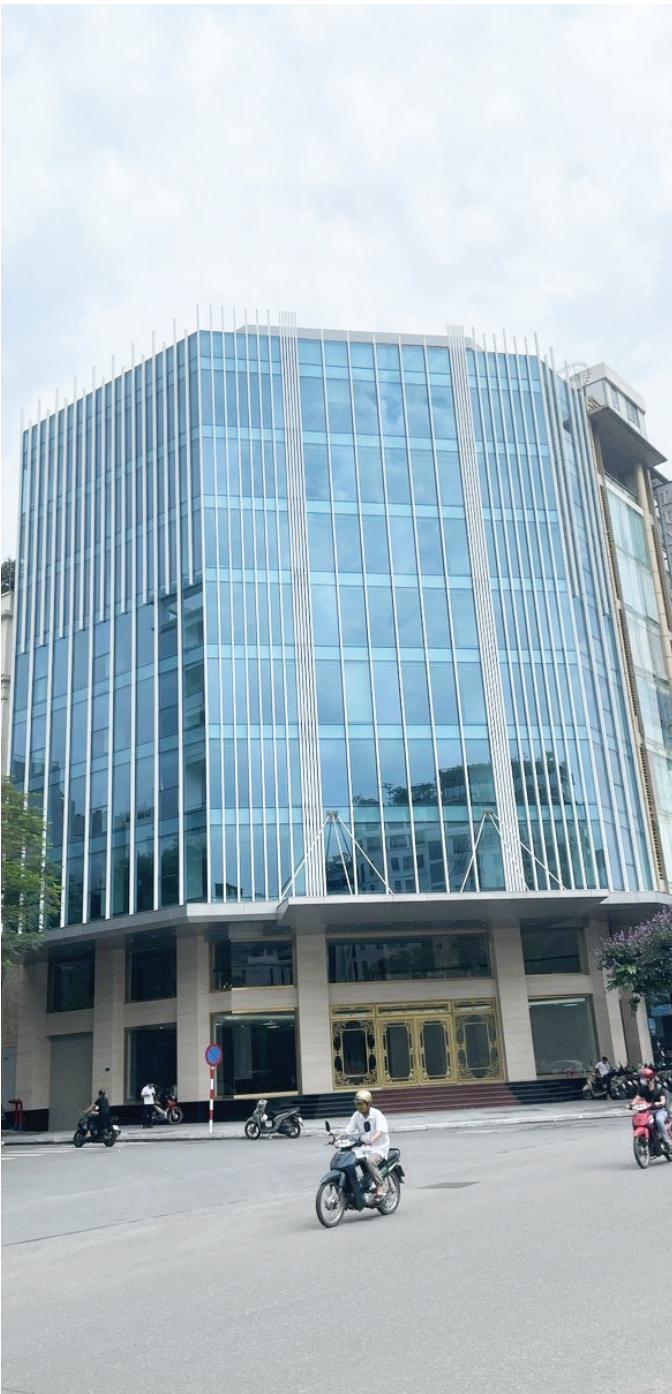
THI CÔNG LẮP ĐẶT HỆ THỐNG PCCC Construction and installation of Fire prevention & firefighting system
